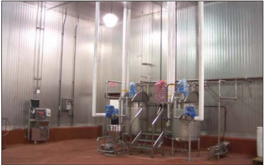
Recipe-based brine mixing system includes a dry ingredient vacuum feed system and ammonia jacketed tanks with a PLC to control transfer pumps and mixing. Source: VCP&A.
